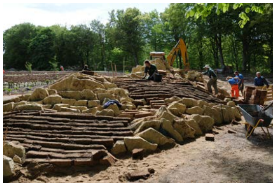
Building the Bangsbo Crevice Garden
